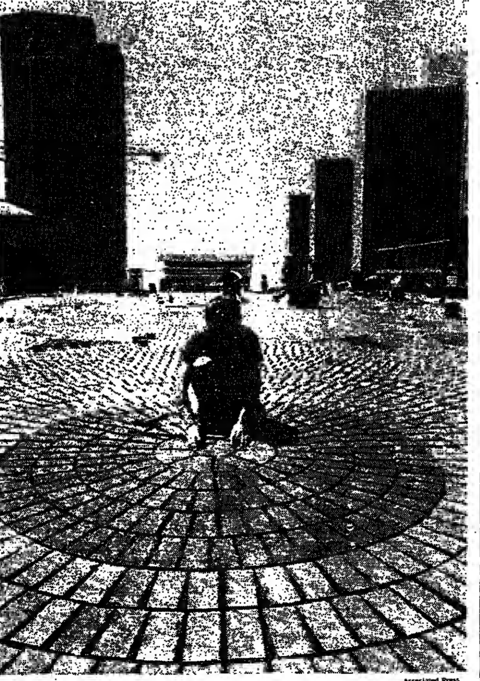
WORK ON THE MALL CONTINUES: Joseph Ghalagher adjusting the center piece of a brickwork geometric design on the south mall of the Empire State Plaza in Albany yesterday. The view is south from the Capitol with the Tower and unfinished Meeting Center at left, the Cultural-Education Center at center, and agency buildings at right.
